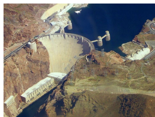
2 GIGAWATTS = 2,000,000,000 WATTS Peak output of the Hoover Dam
